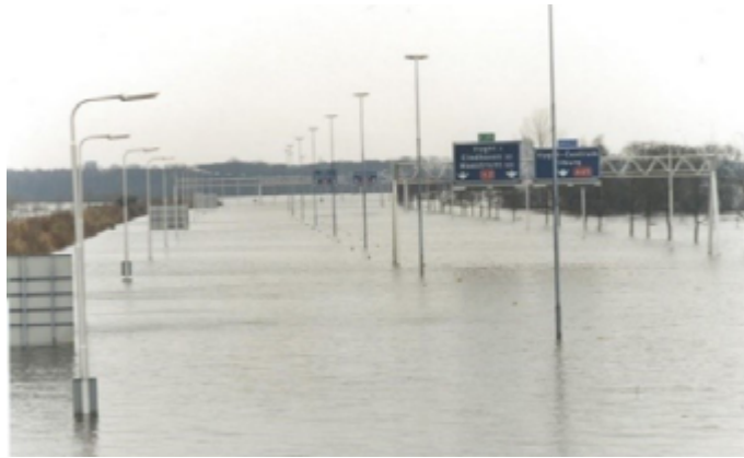
Figure 2. Example of fluvial flooding risks: High water events in 1995 and in 2005 caused a major dike burst near the city of Den Bosch (30 km south of Utrecht), causing the highway A2 to be flooded for multiple weeks. Source: Dutch Ministry of Infrastructure and Water Management, 2005.
